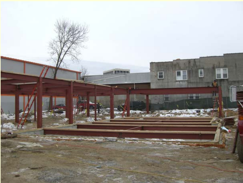
Super Structure January 2009
