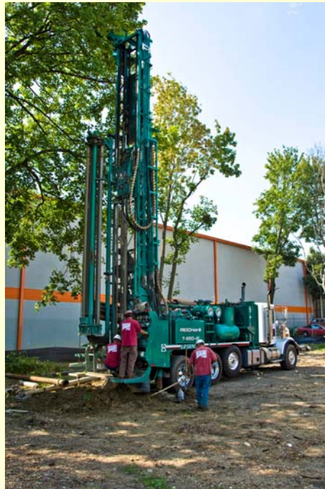
Geothermal Well Drilling August 2008
