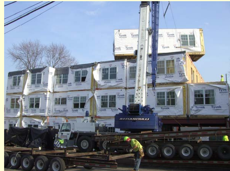
Unit Installation February 2009
